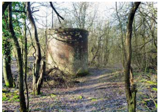
One of the shaft tops, probably shaft 4 or 5. Shaft 3 was sunk in steeply sloping ground which would have been difficult for access for supplies and a difficult location for the stationery steam winding engine which probably operated at that location. Photo by Robin Webster. Reproduced from Geograph under creative commons licence
